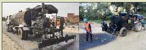
BITUMEN / EMULSION SPRAYER
