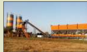
CONCRETE BATCHING PLANT
